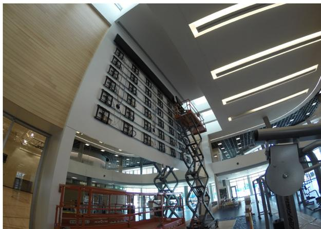
One of the challenges of providing this solution was the space designated to house equipment. Many of the components had to be assembled and prepared a far distance from the actual wall, using remote power supplies. To reduce weight and spatial constraints, the power supplies were also pulled out of the displays and rack-mounted along with media players in a separate, temperate-controlled room with low voltage cables running to the displays
